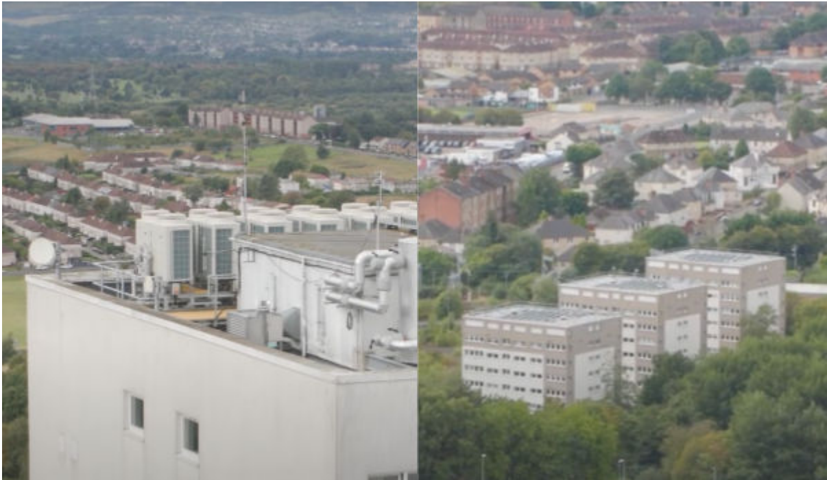
Figure 12: Roof mounted ASHPs at Balgrayhill and solar PV on the Carron Estate
