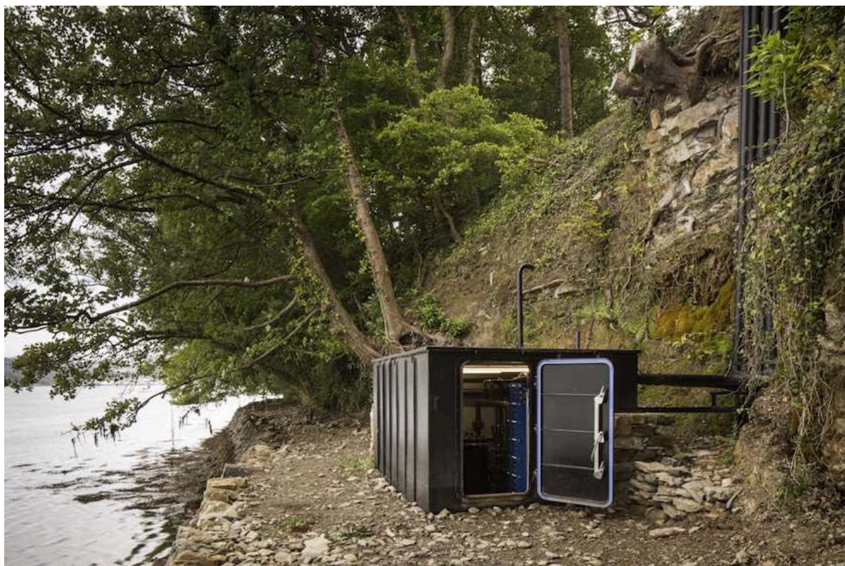
Figure 10: Plas Newydd House, sea water heat exchanger and pump house 34
