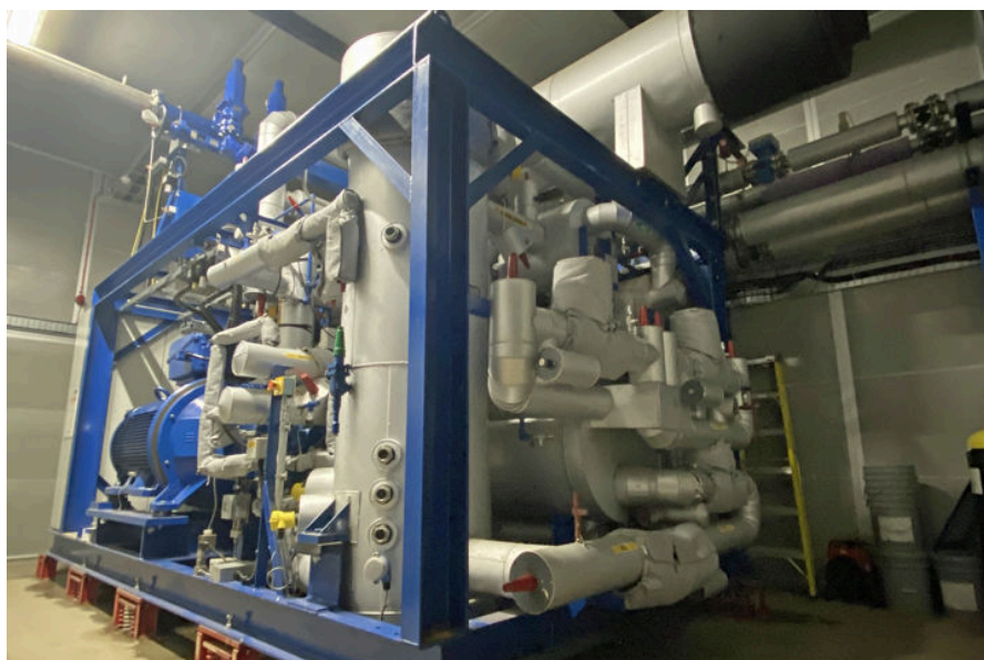
Figure 4: 700kW water source heat pump used in the Viking Heat Network
