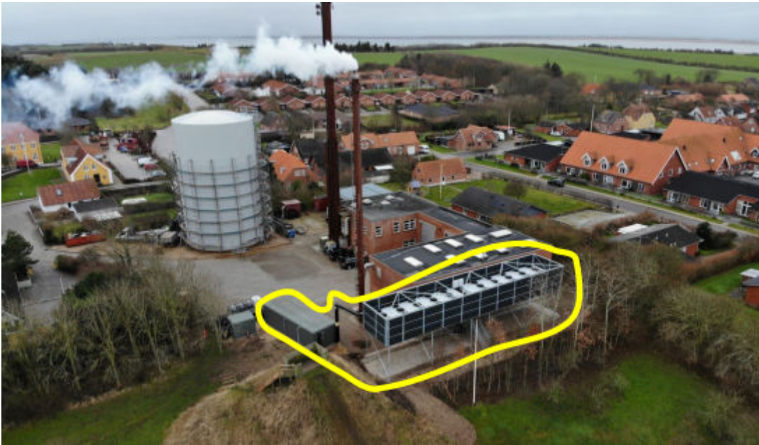
Figure 16: Vestervig Fjernvarme 24 1.2MW ASHP (highlighted) and biomass energy centre
