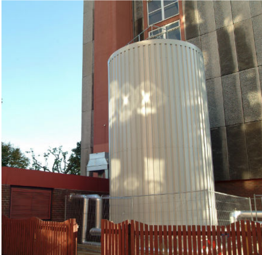
Figure 17: Example of a thermal store
