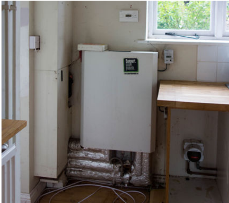
Figure 20: HIU located in a property
