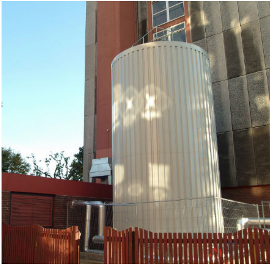
Figure 11: Example of a thermal store
