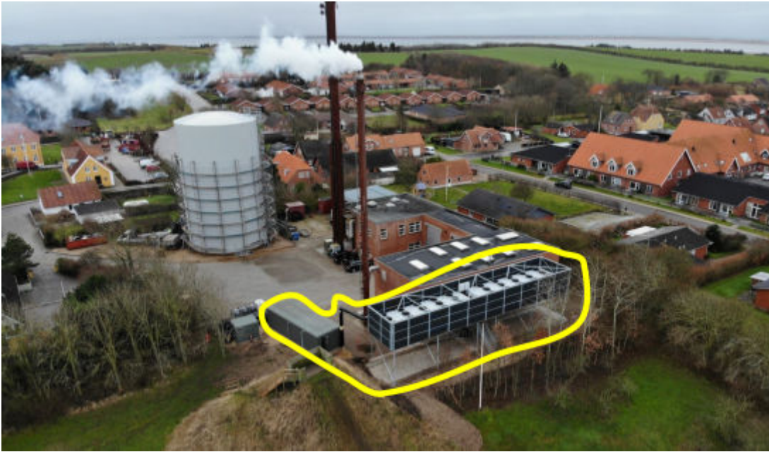
Figure 13: Vestervig Fjernvarme 21 1.2MW ASHP (highlighted) and biomass energy centre
