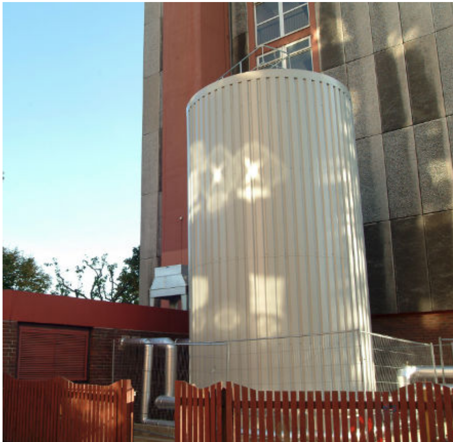
Figure 14: Example of a thermal store
