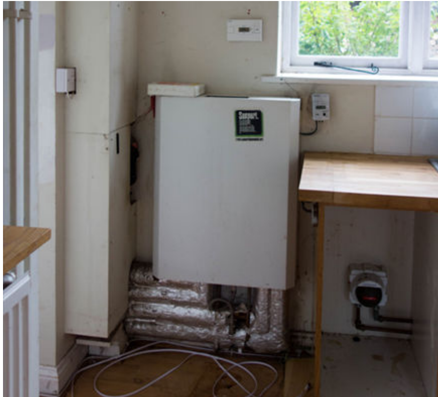
Figure 17: HIU located in a property
